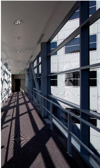
Figure 8.2: Fixed windows in corridor
